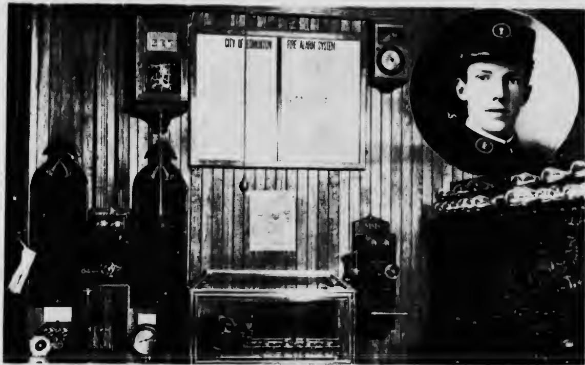
CENTRAL STATION EQUIPMENT OF FIRE ALARM SYSTEM R. W. BRODER FIRE DEPARTMENT ELECTRICIAN
